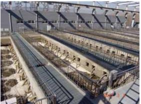
used for wastewater treatment. Technical indicators: new technologies such as gas impulse and mechanical cleaning are integrated into the membrane unit; a variety of techniques controlling the filterability of the mixed liquor enable the extension of the membrane operation cycle by 2-4 folds; online chemical cleaning modes are suitable
